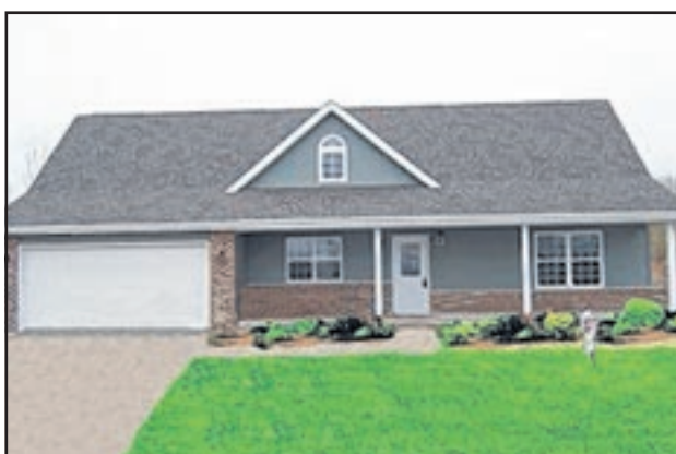
THE WESTFIELD BY HOMES OF THE 20TH CENTURY: 1951 Westfield, Griffith, 1 1/2 story single family home, 2,170 square feet, four bedrooms, two baths. Win this home and a $60,000 cash prize, based on builder's estimated home value.
